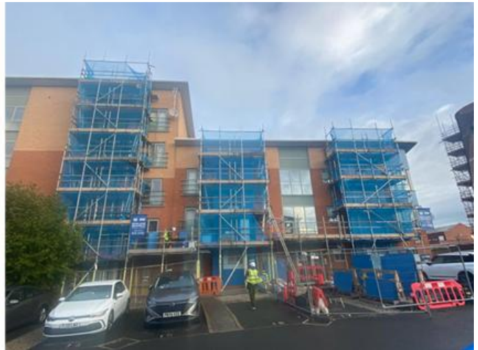
A Photo Showing Panel Installation Has Began
