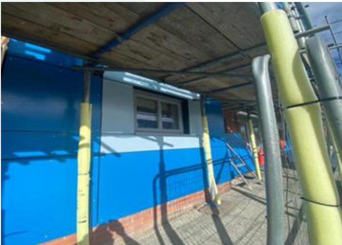
Progression on C2
