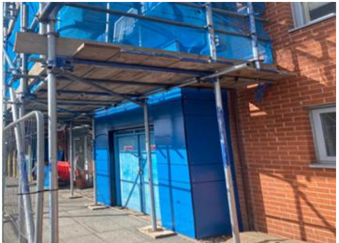
Progression on C3
