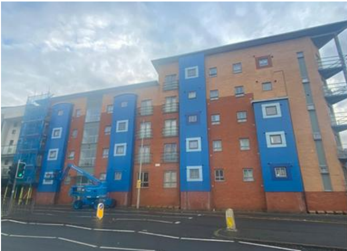
A photo showing Elevation With Panels Installed
